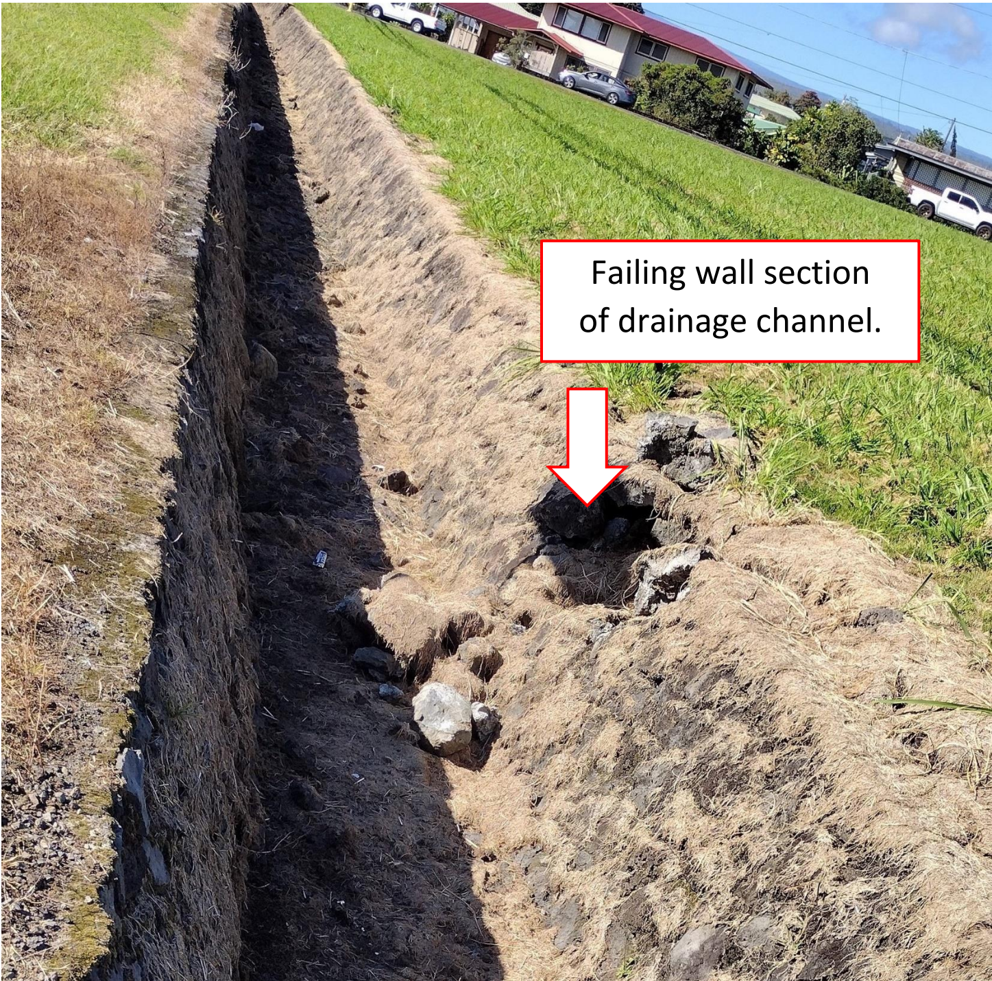
Failing wall section within Drainage Channel.
